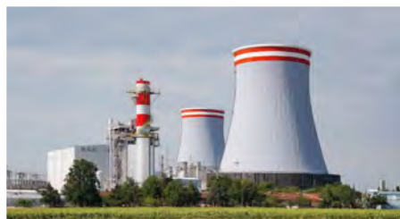
2 x 600 MW CCGP Hamitabat, Turkey, 2017 Natural draft dry cooling tower, DC jet condenser, Heller IDCT
