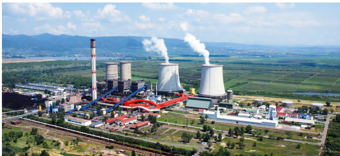
FGD-in-tower in the 800 MW Mátra power plant, Hungary
