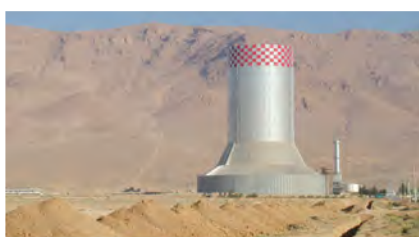
510 MW CCGP Al Nasserieh, Syria, 2008 Natural draft steel structure dry cooling tower, DC jet condenser
