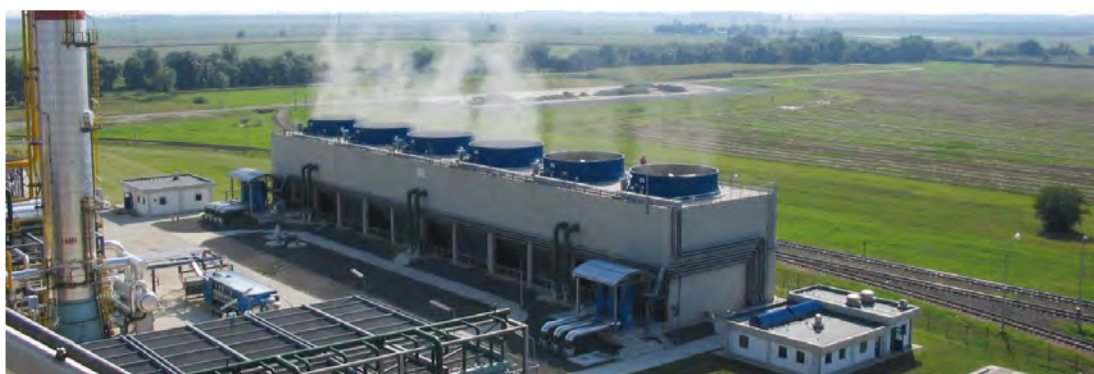
Wet cooling tower, TVK Chemical Works Olefine 2 & HDPE 2 Plant
