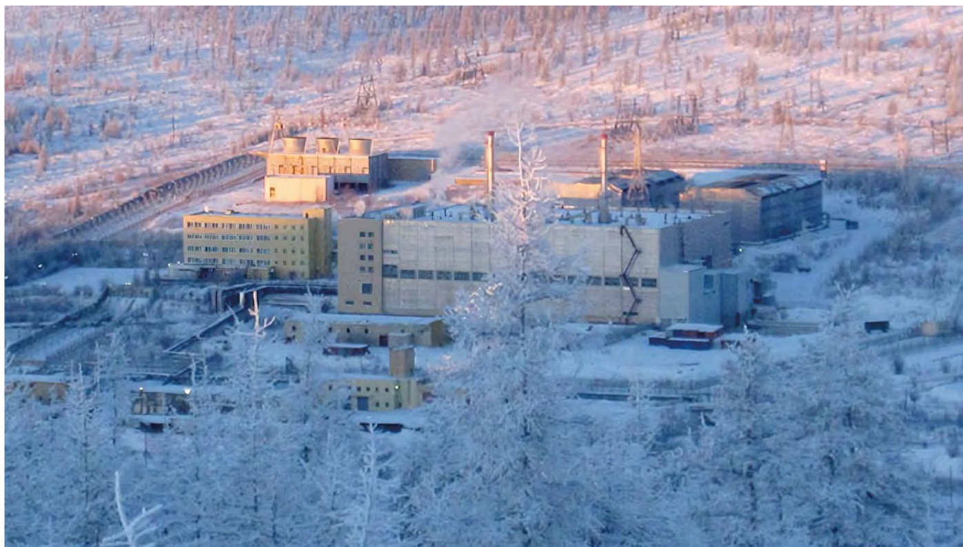
Nuclear Power Station, Bilibino, Russia, Mechanical draft dry cooling tower
