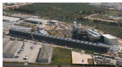
800 MW CCGP Modugno, Italy, 2009 Induced draft steel structure dry cooling tower, DC jet condenser
