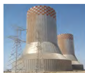
2 x 210 MW CCGP Teshrin, Syria, 1993 Natural draft steel structure dry cooling tower, DC jet condenser, peak coolers
