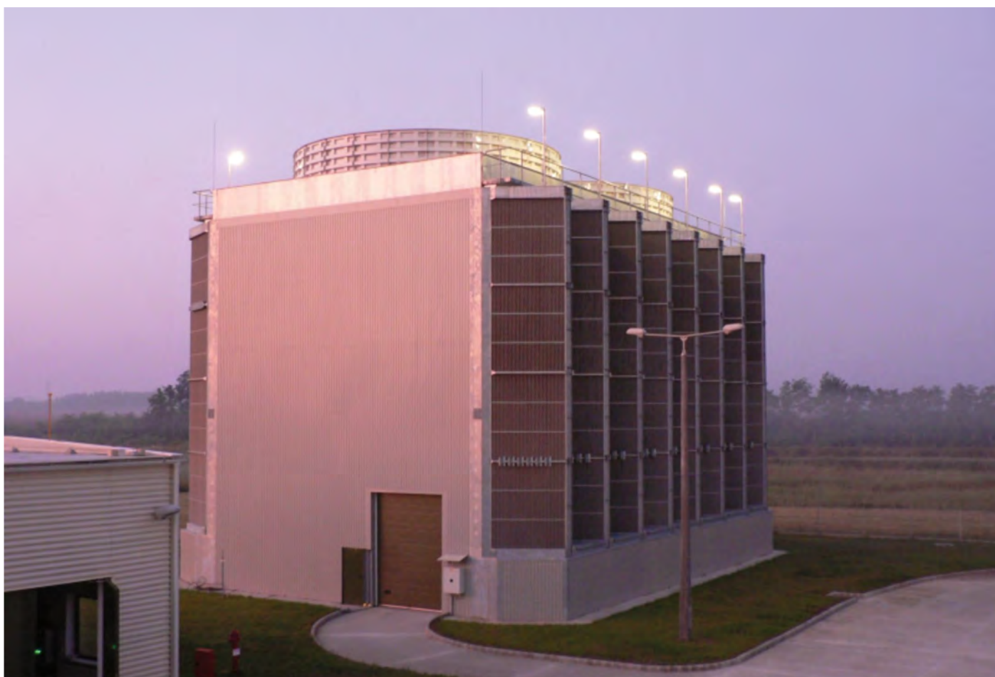
20 MW Biomass Powerplant, Szakoly, Hungary,
