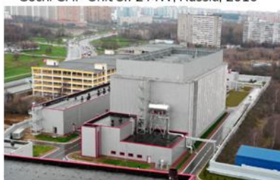
Induced draft steel cooling tower with supplementary spraying Sochi CHP Unit 3.72 MW, Russia, 2010
