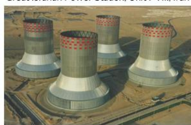
Natural draft steel structure dry cooling tower, DC jet condenser, peak coolers Great Isfahan Power Station, Unit I-VII., Iran
