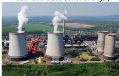
Natural draft dry cooling tower, DC jet condenser Mátra Power Station, Unit IV, Hungary
